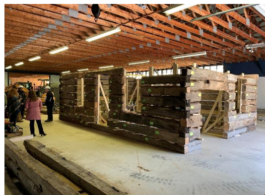
Figures 4 and 5 – The cabin puzzle was reassembled by ‘dry fitting’ the loose logs inside one of the large agricultural exhibition buildings at Lambton Heritage Museum. Once reviewed by the architect, the cabin was again taken apart and stabilization work undertaken on the logs.
