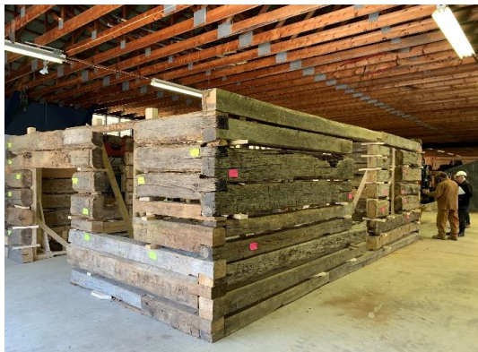
Figures 4 and 5 – The cabin puzzle was reassembled by ‘dry fitting’ the loose logs inside one of the large agricultural exhibition buildings at Lambton Heritage Museum. Once reviewed by the architect, the cabin was again taken apart and stabilization work undertaken on the logs.
