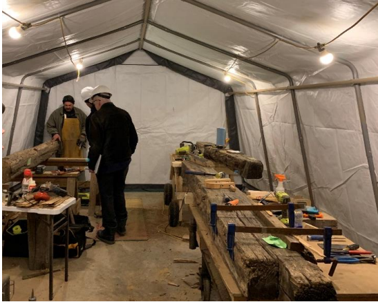
Figure 6 – Logs with evidence of rot and deterioration that could be salvaged for use were treated and filled with a concealed epoxy to prevent further degradation.
