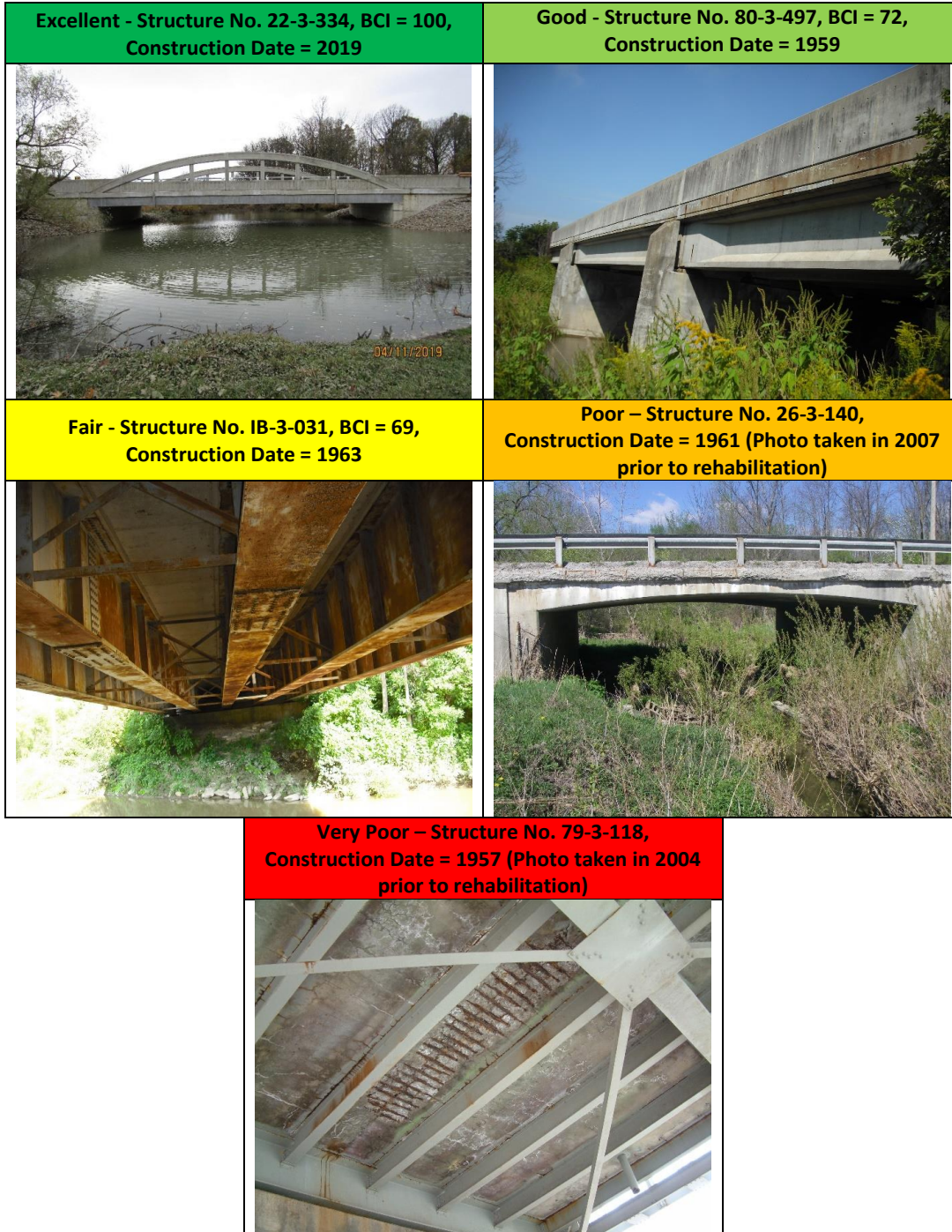
Figure 3-4: Local Examples of Bridge Condition
