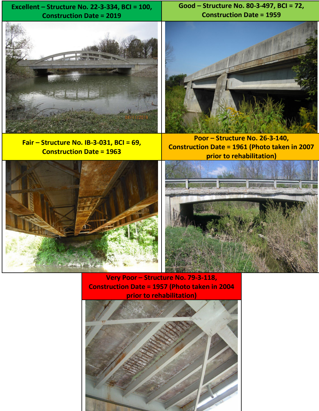
Figure E-4: Local Examples of Bridge Condition
